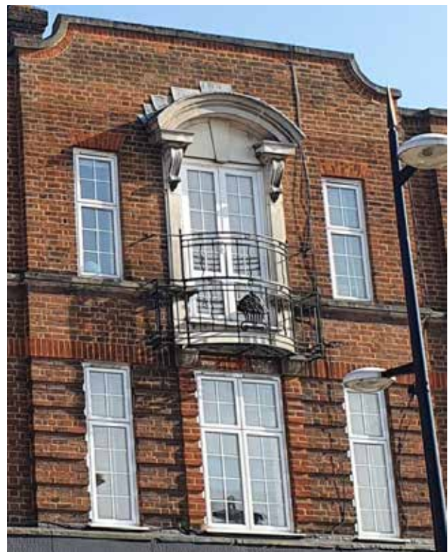
View of one of the 'gabled' sections of the main elevation to the existing building showing the detailed brickwork, stone pediments and decorative steel Juliet balcony
